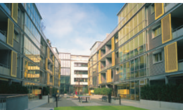
Akazienhof housing development, Zurich, Switzerland.
